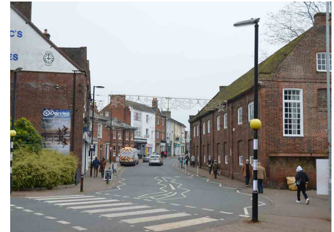
Figure 08: Bridge Street leading to Leighton Buzzard High Street.
