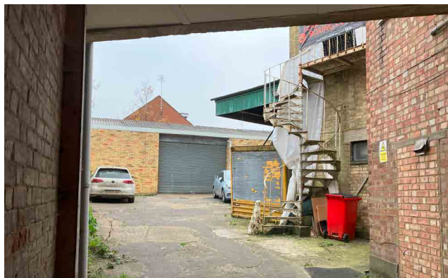
Figure 57: Potential site for redevelopment, 3 Market Court, Hockliffe Street.
