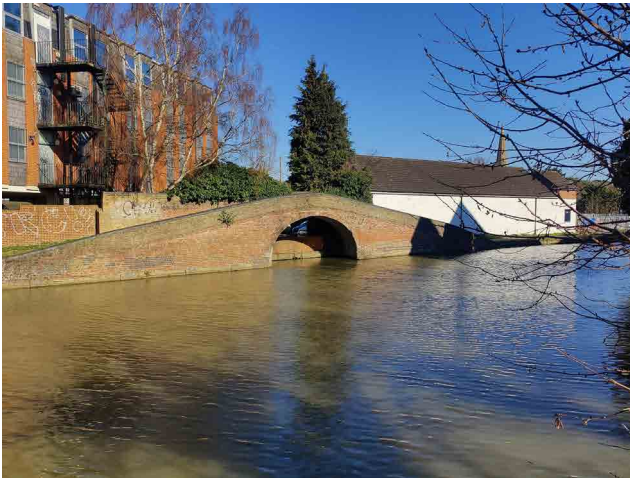
Figure 71: Former entrance to the old canal basin.
