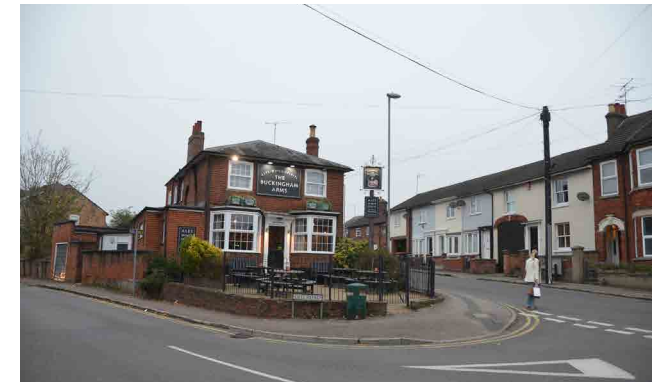
Figure 67: High quality corner building and public house, The Buckingham Arms pub.
