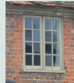
Timber sash window
