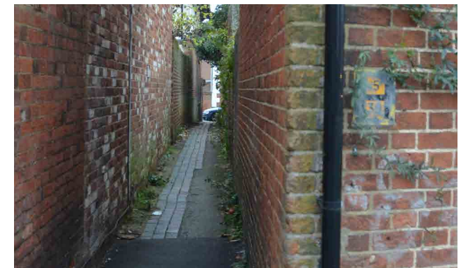
Figure 68: Some retained historic blue bricks along a footpath between buildings in Linslade.
