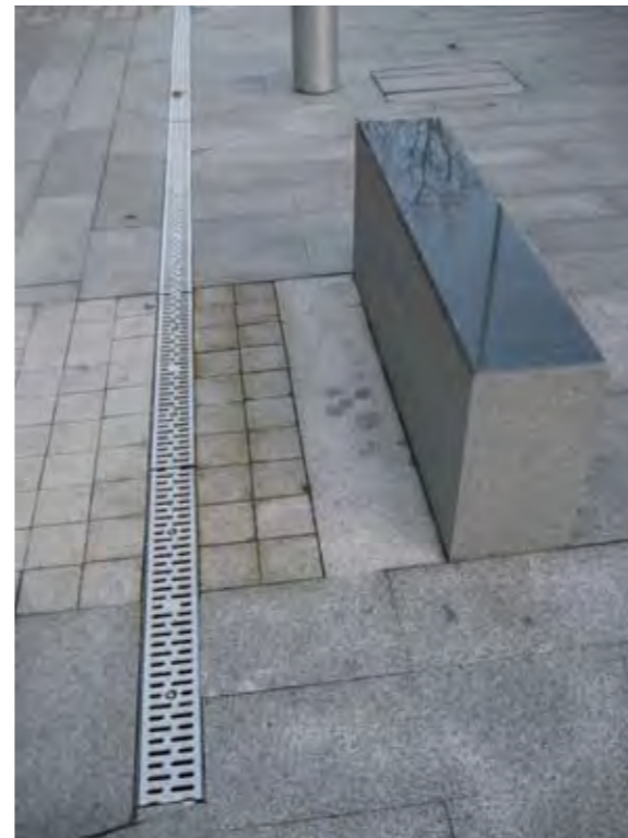
FIG. 7.4 Tower Bridge Road, London
