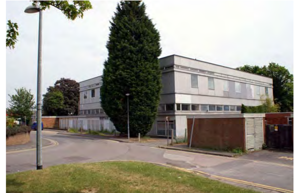
FIG. 2.8 Telecoms building adjacent to the site on Duncombe Drive
