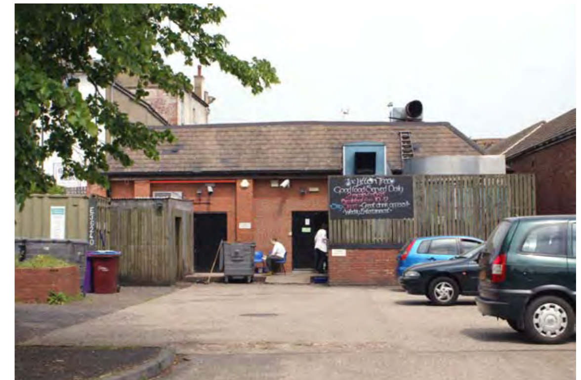
FIG. 2.6 Service access to the Litten Tree pub from Duncombe drive
