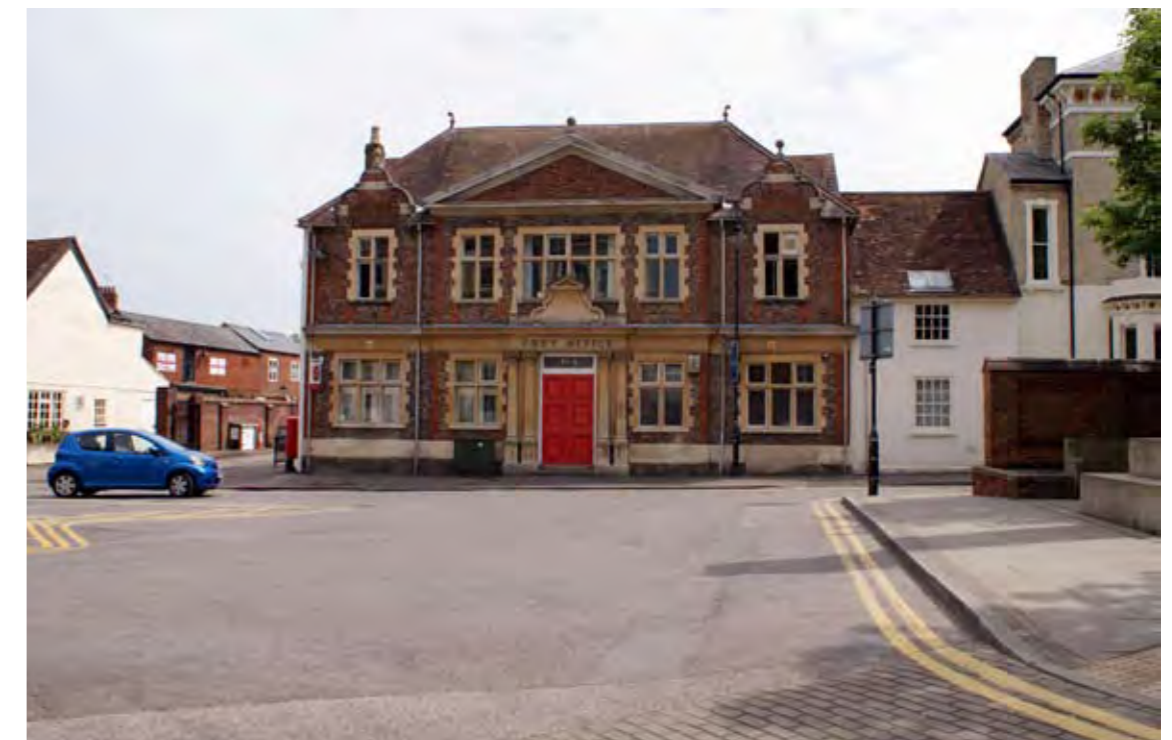
FIG. 2.16 The old Post Office, formerly a school
